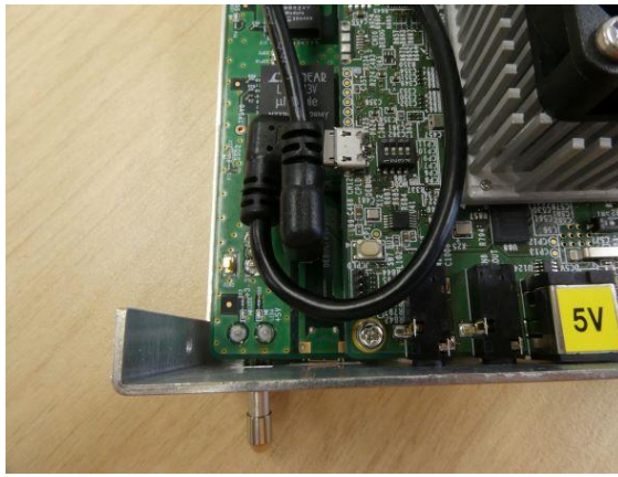
Picture 6-7 example of cable connection (top)
